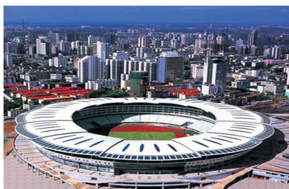
Completion of the WNIC office inside HeLong Stadium
